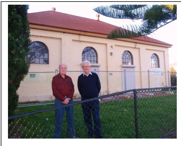
Photo: Ernie Johnson and Colin Mondy outside Winder House where restoration work has started.
