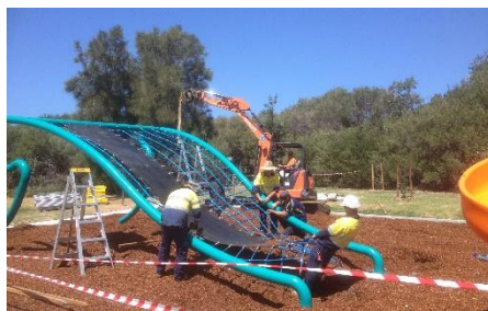
Wave-shaped climbing frame under construction
